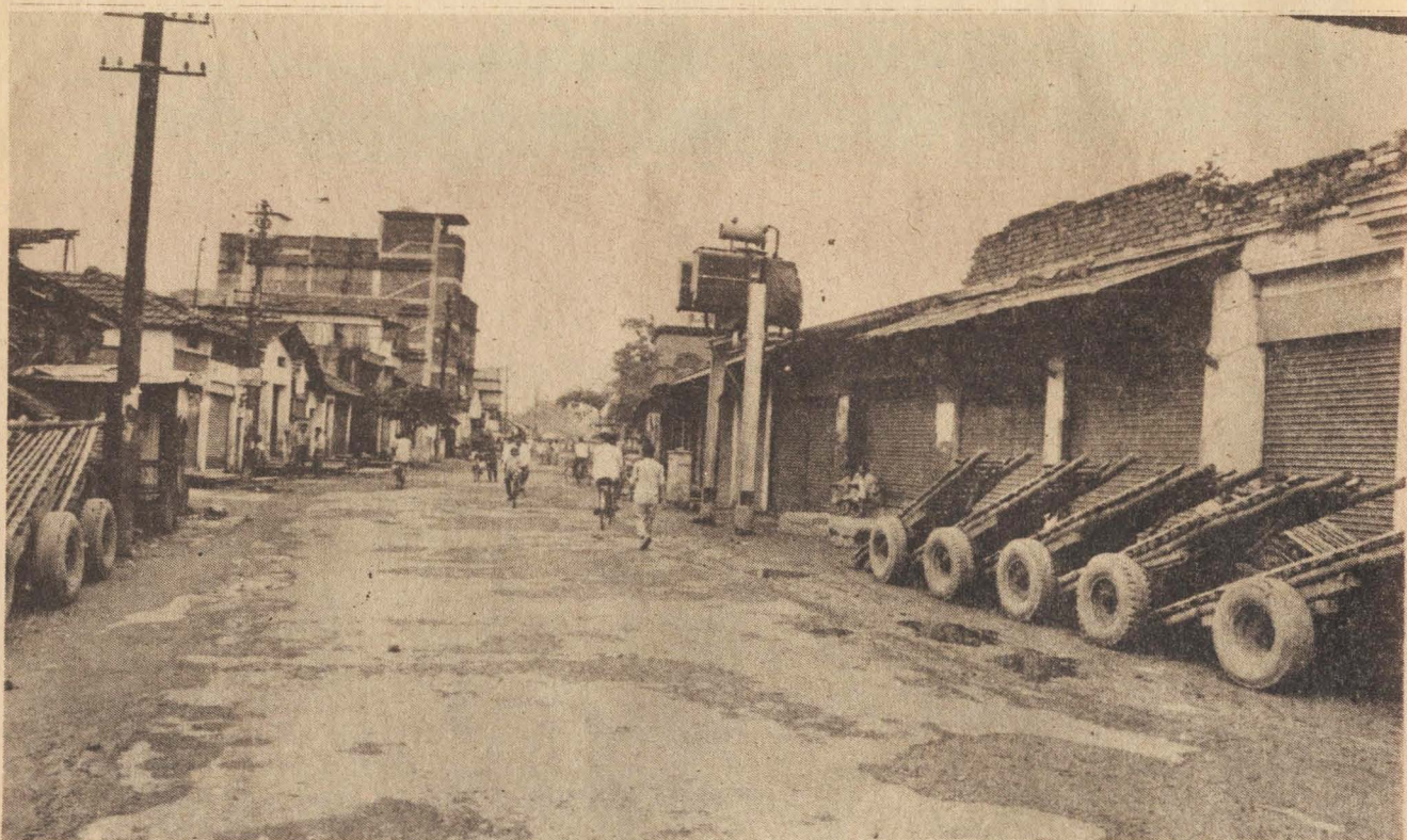
Balilas Road, Howrah, a busy small scale Industrial Sector totally closed.
